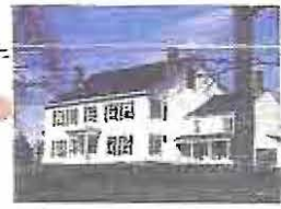
Philip Van Horne House Gen. William Alexander, Lord Stirling stayed here. 941 East Main Street Bridgewater, NJ 08807
