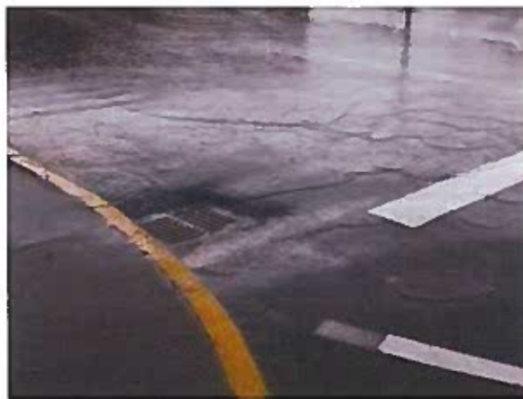
Figure 1: Stormwater draining from a parking lot
